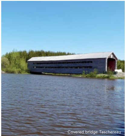
Covered bridge Taschereau
