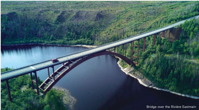
Bridge over the Rivière Eastmain
